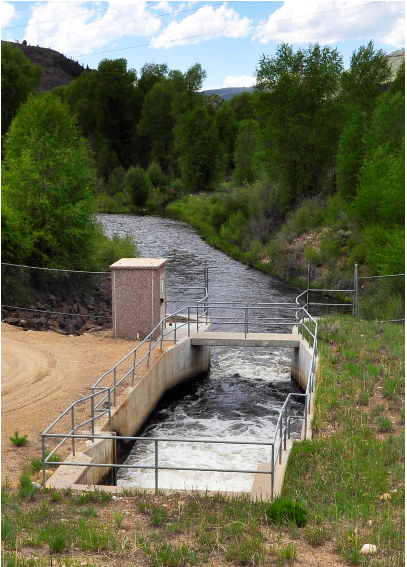
This bypass outlet structure at Windy Gap Reservoir allows for required water releases into the Colorado River.
